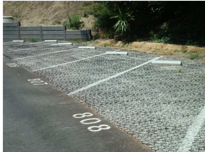
Permeable paving allows stormwater to filter through the surface of parking lots, improving water quality and reducing runoff handled by storm drains
