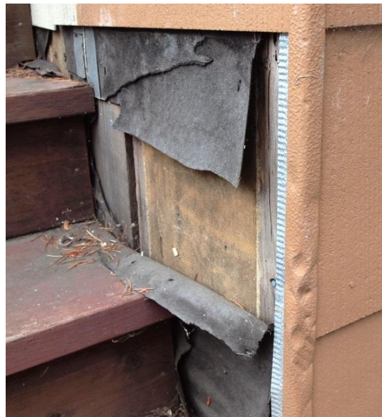
Detail of vertical board-and-batten siding beneath current siding at water tower.
