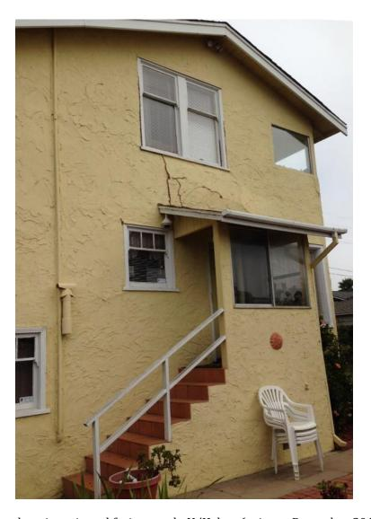
Rear elevation, viewed facing north; U/K date (prior to December 2014) By Tim Martin  $\underline{\text{NOTE}} : \text{Stucco damage and aluminum wind break at porch}$
