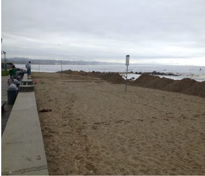
Figure 14. Berms built at Capitola Beach help to decrease coastal flooding of the Village (Photo: R. Clark)
