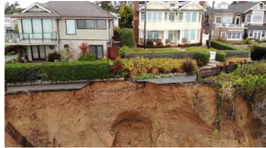
Figure 12b – Grand Avenue Pedestrian Pathway Erosion
