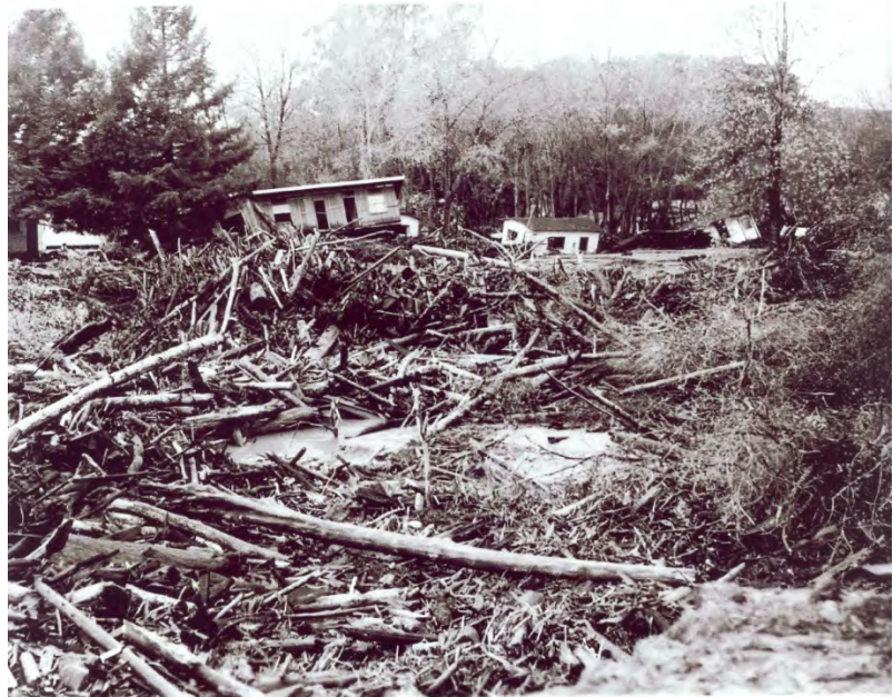
Figure 15 - Debris generated during the Flash Floods (ca. 1955)
