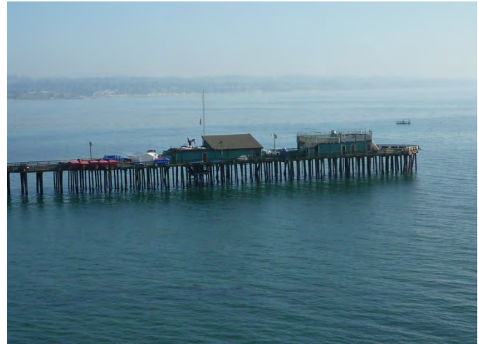
Figure 5 - View of Capitola Wharf looking South (ca. 2012)
