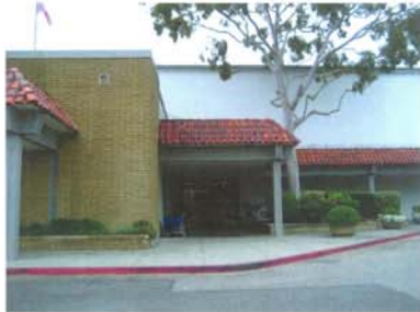
EXISTING SEARS ENTRANCE
