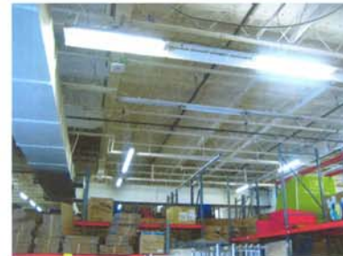
UNDERSIDE OF EXISTING DECK
