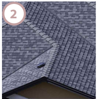
Composition Shingle Roofing
