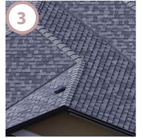
Composition Shingle Roofing
