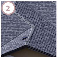
Composition Shingle Roofing
