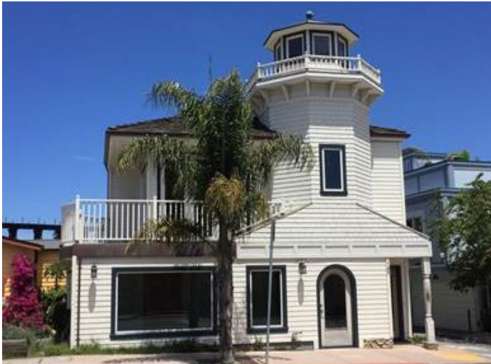
Example of enhanced building design at intersection corner at Riverview Drive and Stockton Avenue. The Capitola light house is an iconic building in the central village. Increased height, articulation, and distinctive design creates a strong and informative element in the overall development framework.
