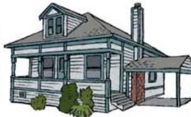
34 Woodhouse House, c1910 104 Fairview Ave.
