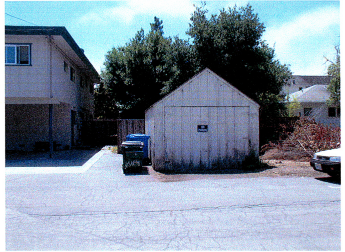
20 – Garage on Project Site (to be demolished)
