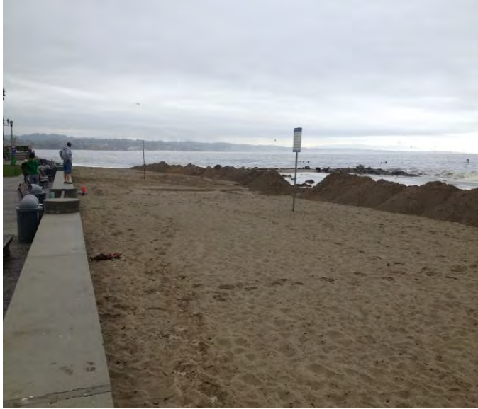
Figure 14. Berms built at Capitola Beach help to decrease coastal flooding of the Village (Photo: R. Clark)
