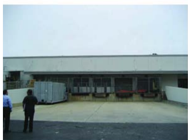
EXISTING LOADING DOCK
