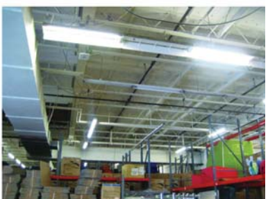
UNDERSIDE OF EXISTING DECK
