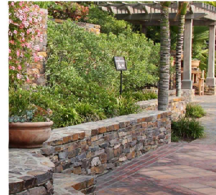
SAMPLE LEDGER STONE SEAT WALL (CAP WOULD NOT BE STONE; WE SUGGEST CAST IN PLACE CONCRETE, DETAILED WITH NOTCHES TO PREVENT SKATEBOARDING)
