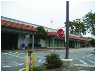
EXISTING SEARS, FUTURE TX
