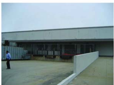
EXISTING LOADING DOCK
