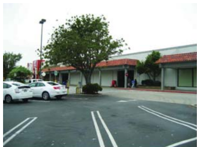
EXISTING SEARS, FUTURE TX
