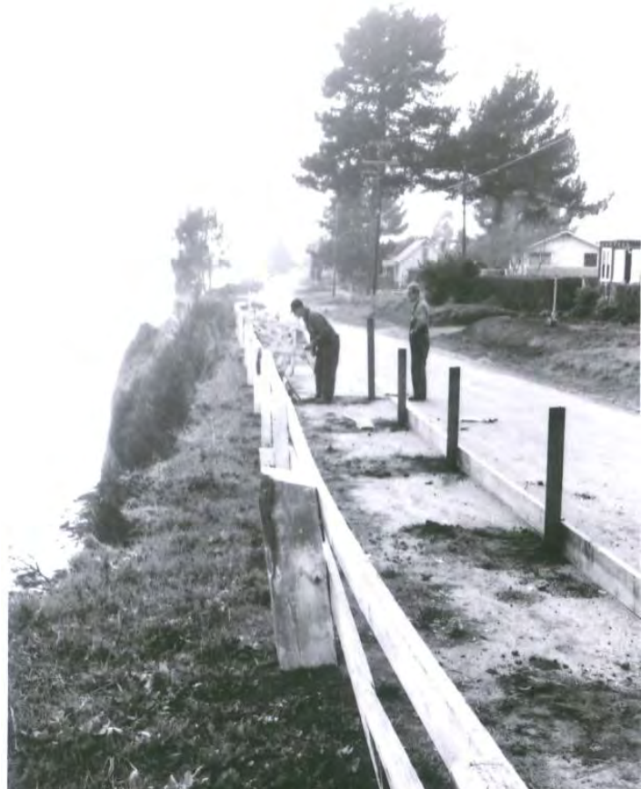
Figure 14 - Bluff Failure along Grand Avenue (associated with 1960 coastal storm)
