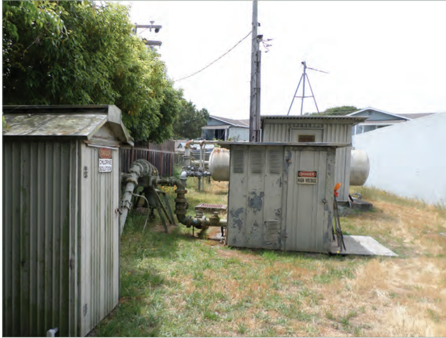
Before Site looking east, as viewed from within perimeter fencing.
