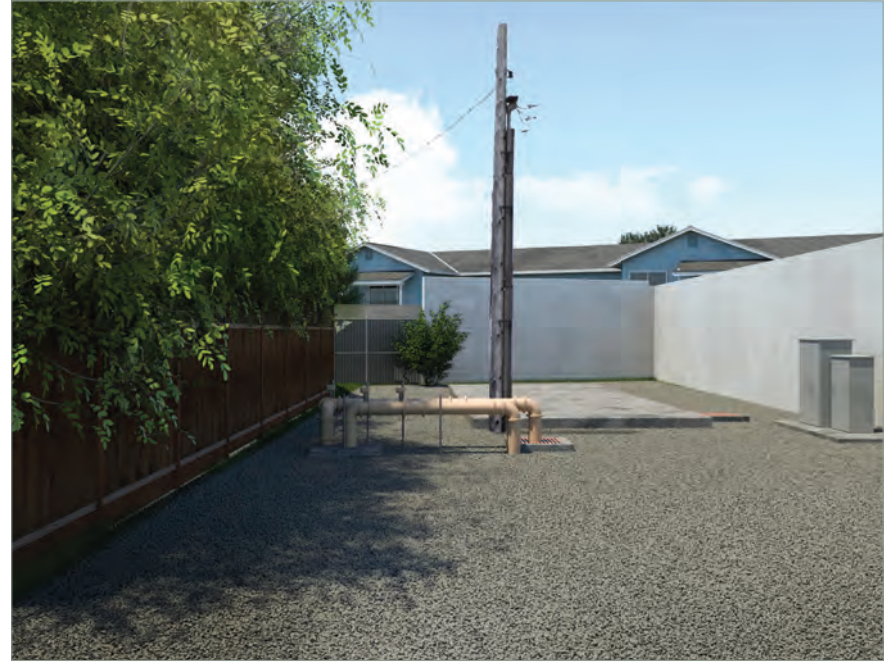
After Site looking east, as viewed from within perimeter fencing. Removal of all above ground structures, piping and treatment vessels. Concrete vault pad remains. Addition of recharge well and backwash pump along with motor control center. Vegetation cut back and introduction of gravel.
