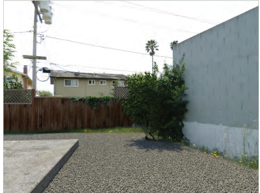
After Site looking south, as viewed from within perimeter fencing. Removal of all above ground structures, piping and treatment vessels. Concrete vault pad remains.
