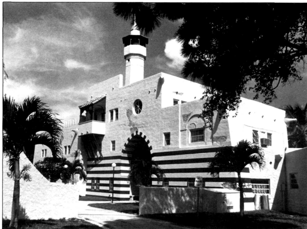
Opa-Locka Company Administration Building, Opa-Locka, Florida: anchor building for planned city conceived by inventor and real estate developer Glenn Hammond Curtiss (Mary Evans).
