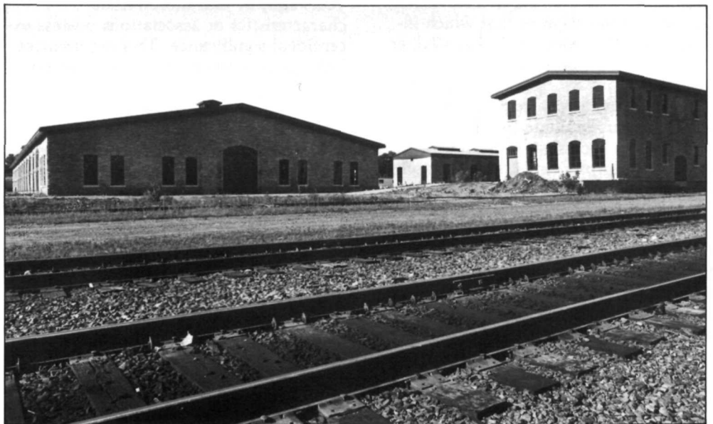
St. Paul, Minneapolis, and Manitoba Railway Company Shops, St. Paul, Minnesota (Miller F. Dunwiddie).
