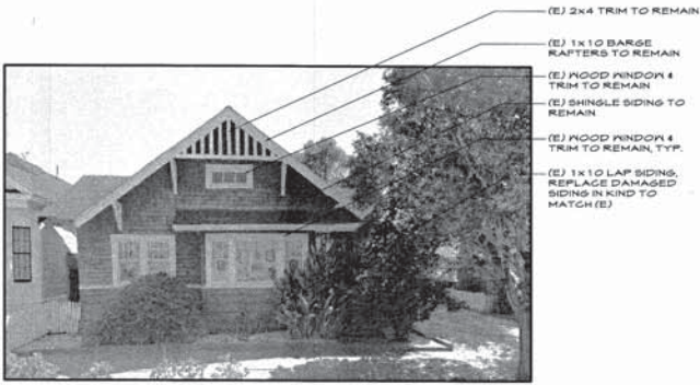
1 EXISTING FRONT ELEVATION - RESIDENCE SCALENONE
