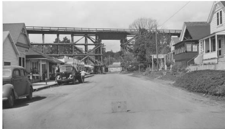
Historic trestle crossing Capitola Avenue
