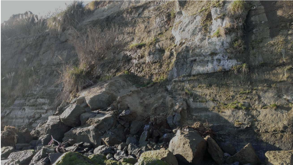
Coastal Bluff Erosion Debris on Beach as it Existed on November 7, 2014 at the Property
