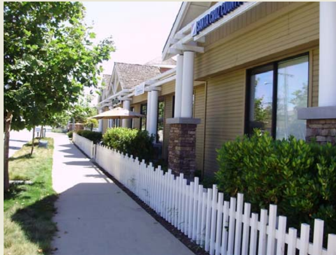
Windows, landscaping, and architectural detail add visual interest to the Nob Hill shopping center on Bay Street
