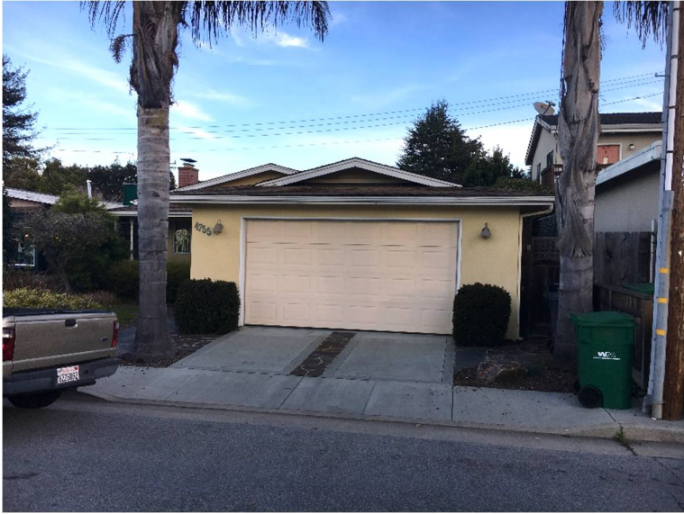
4755 Garnet Street – 10 feet
