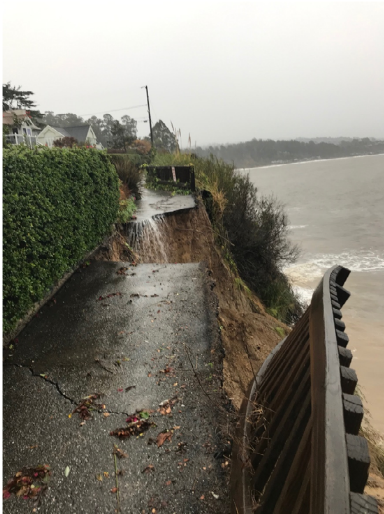
Runoff draining into area of slope failure
