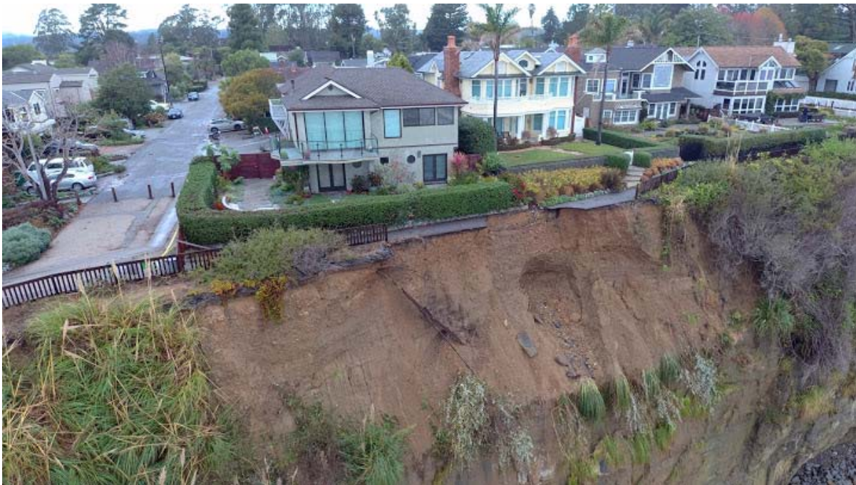
December 4, 2019 drone photo of slope failure along Grand Avenue pathway. Oakland Avenue to the left of photo.
