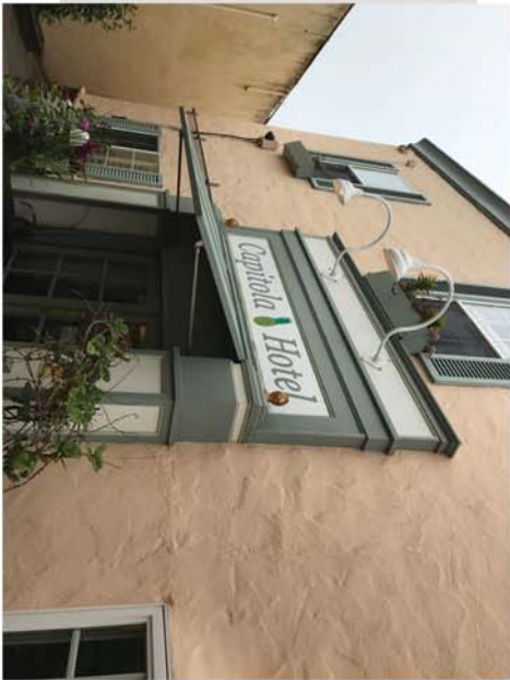
EXISTING EXTERIOR SIGNAGE - COURTYARD LOCATION TO BE REMOVED
