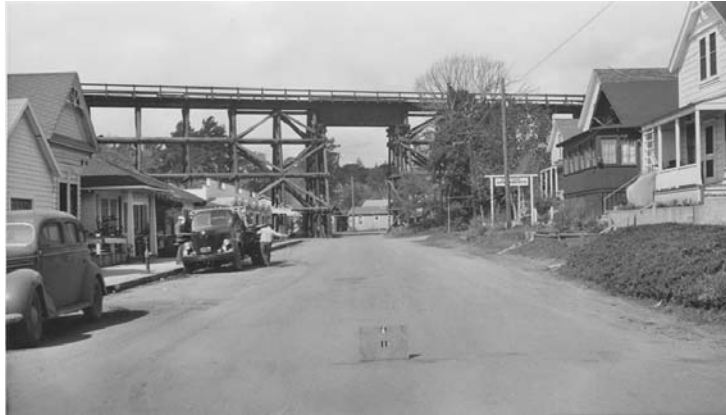
Historic trestle crossing Capitola Avenue
