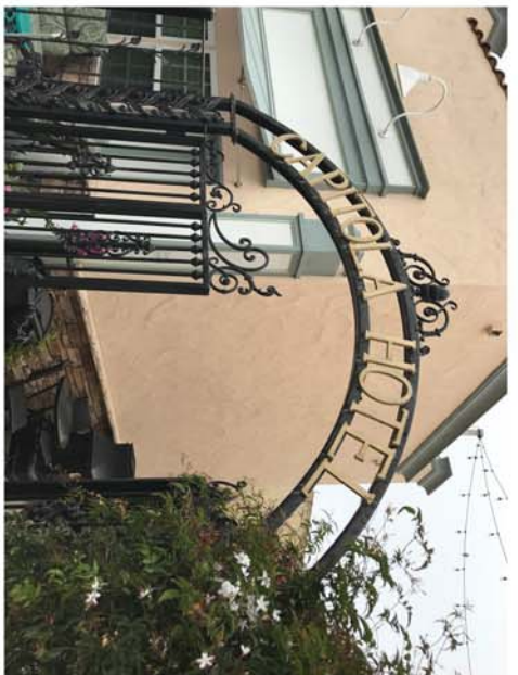
EXISTING ARBOR SIGN AT COURTYARD ENTRY EXISTING TO REMAIN UNCHANGED OVERALL DIMENSIONS: APPROX. 8' WIDE X 12" TALL ON A CURVE
