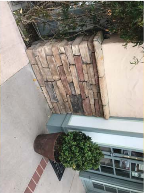
EXISTING STONE FACADE TO REMAIN, PROPOSED PROJECTING SIGNAGE TO BE LOCATED ABOVE EXISTING STONE - EXISTING STONE PROJECTS 4" INTO SIDEWALK SIDEWALK IS 10" WIDE OVERALL PROPOSED PROJECTING SIGNAGE TO PROJECT 4" OVERALL PROPOSED PROJECTING SIGN DOES NOT PROJECT FARTHER THAN EXISTING SIGN.
