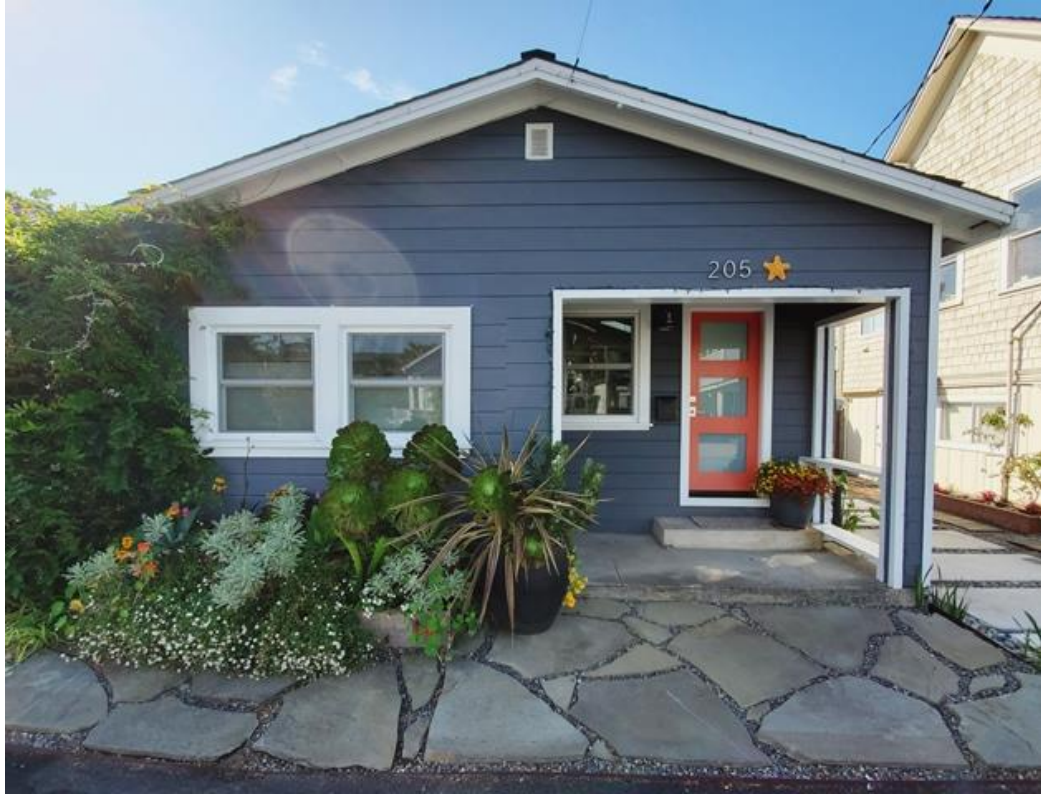
Front Façade. Viewed facing south. May 2020. (Photo by Matthew Orbach, City of Capitola)
