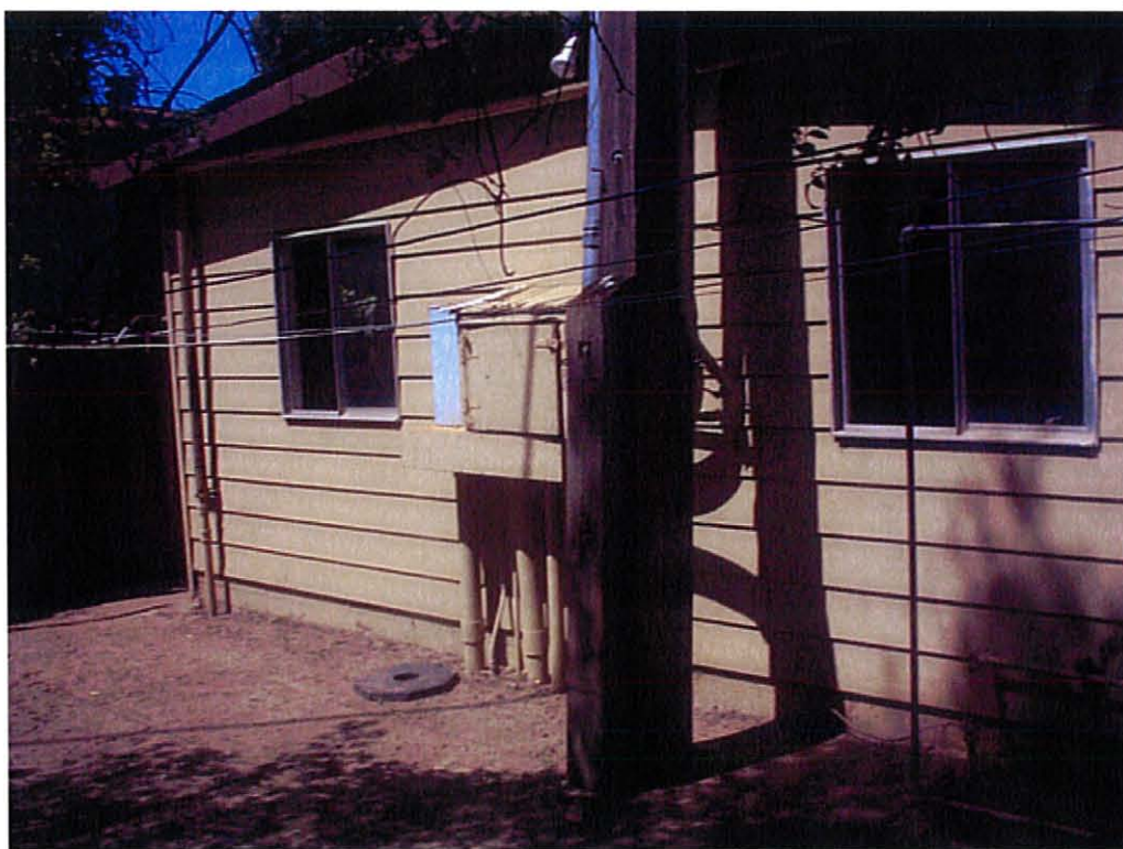
Rear of laundry building
