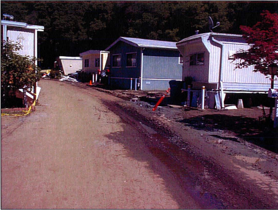
Roadway condition after flooding on 3/26/11
