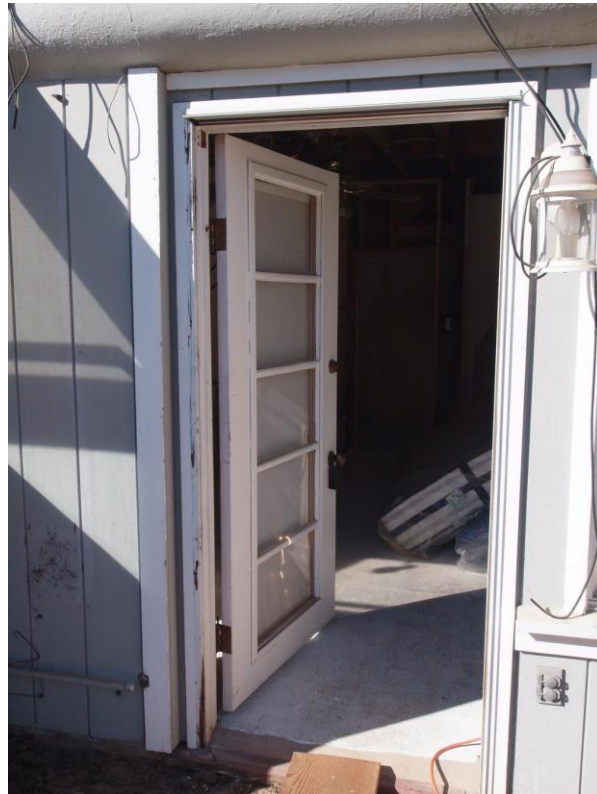
Entry to rear residential unit.
