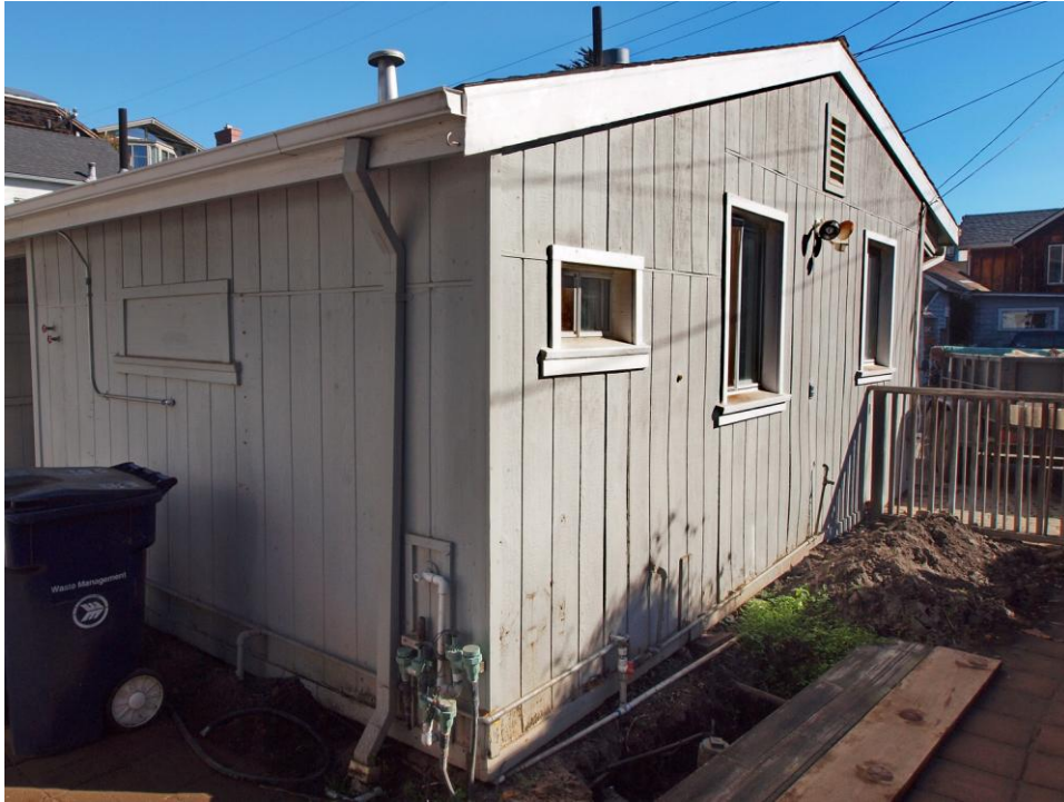
Rear and side west side elevation of cottage.
