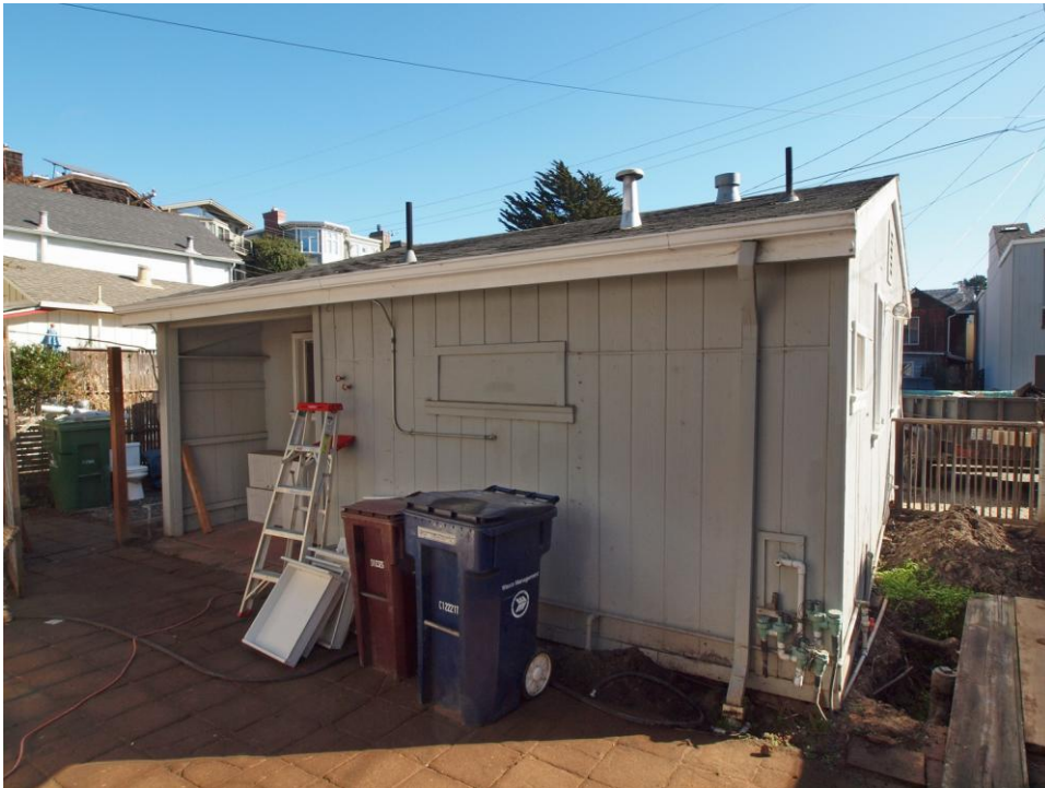
Rear elevation of cottage.
