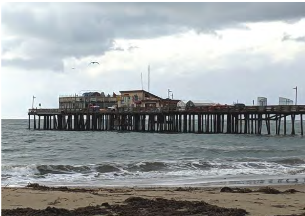
South end of Wharf with Buildings, viewed facing southwest. 12/14/18. Leslie Dill
