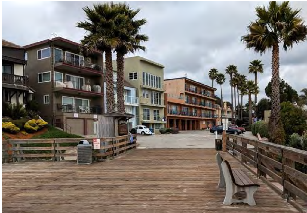
Pier entrance, viewed facing north. 12/14/18. Leslie Dill.
