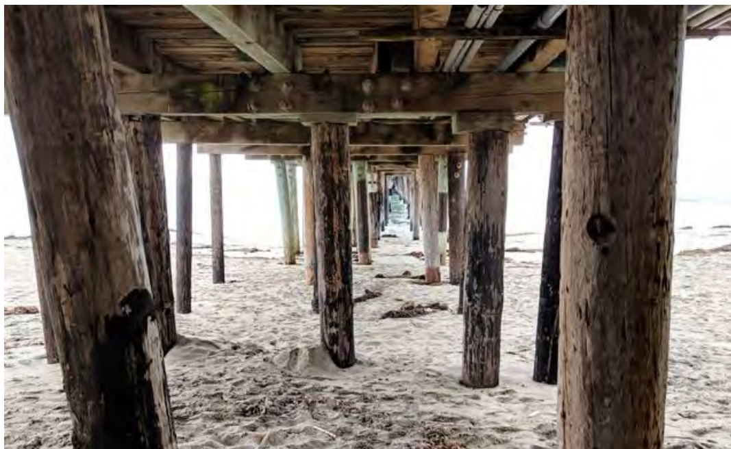
Pilings and girders beneath Wharf, viewed facing south. 12/14/18. Leslie Dill.
