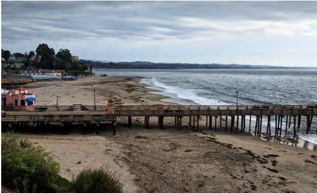
Wharf entrance, viewed facing east. 12/14/18. Leslie Dill
