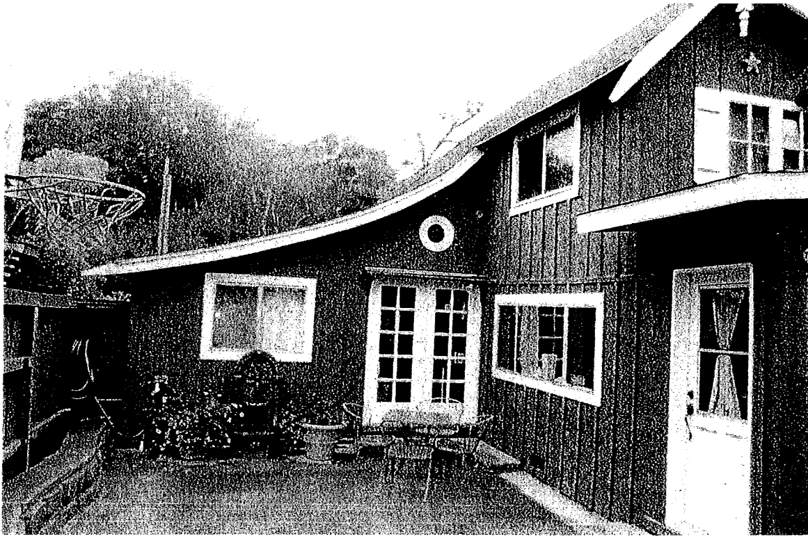
Photo #1. Looking SW at the NE facing facade, September, 2013.
