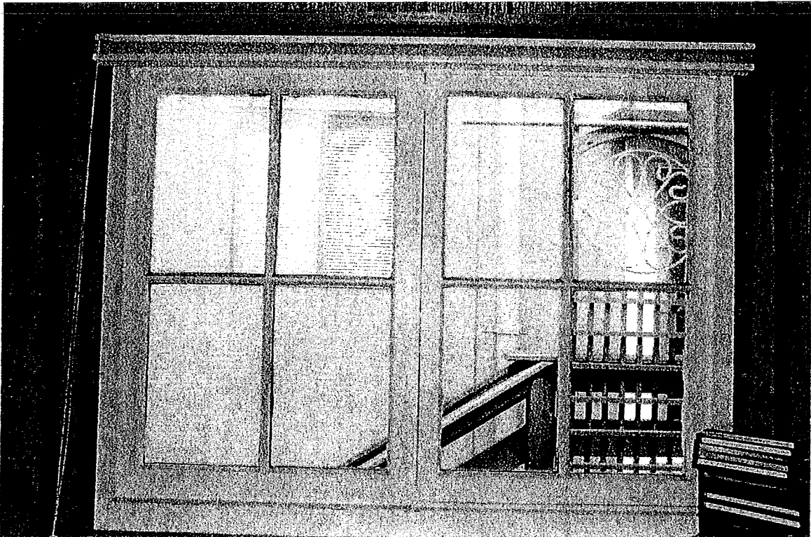
Photo #5. Typical original wood casement windows found along NW side-elevation, Sept., 2013
