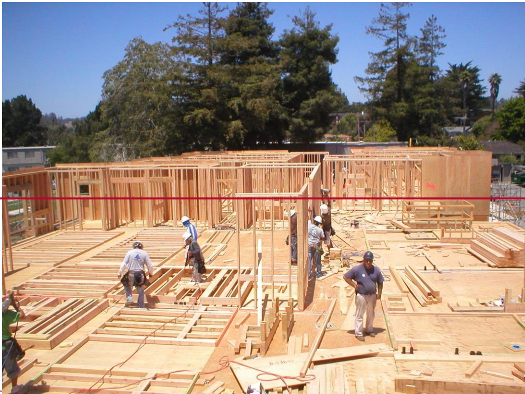
Construction at 750 Bay Avenue
