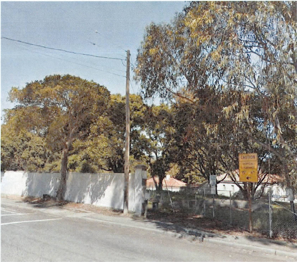
Original Pole - City asked Nexius to move locations due to redevelopment.
