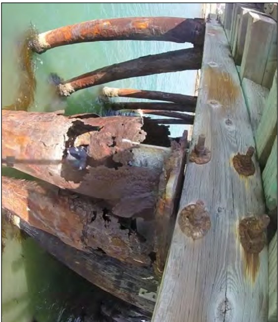
PHOTO 3 STEEL PILES - BENT 76C
