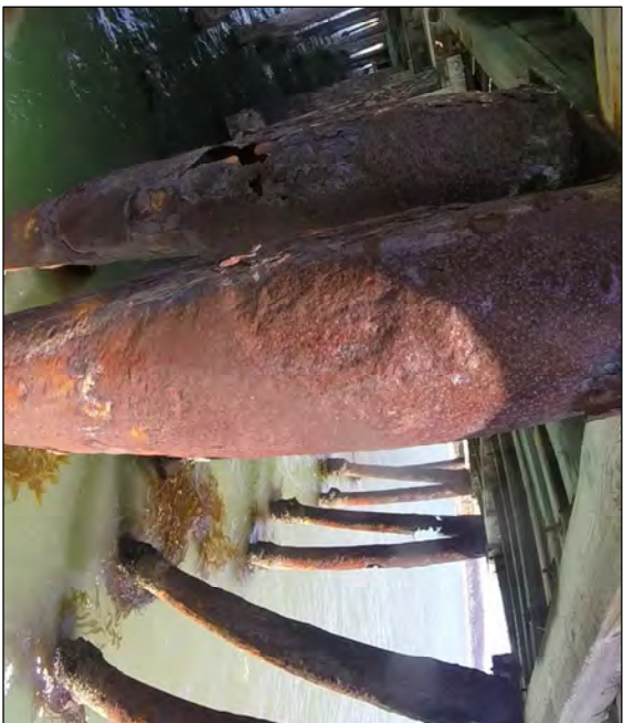
PHOTO 4 STEEL PILES - BENT 76D
