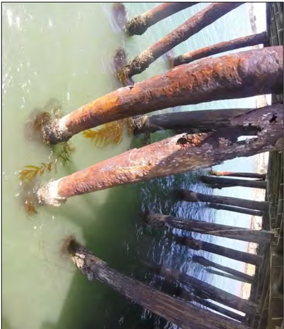
PHOTO 2 STEEL PILES - BENT 75B
