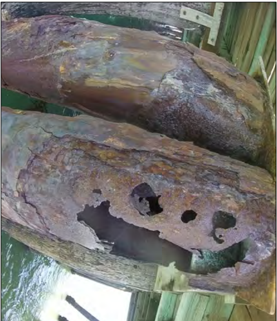
PHOTO 6 STEEL PILES - BENT 75F
