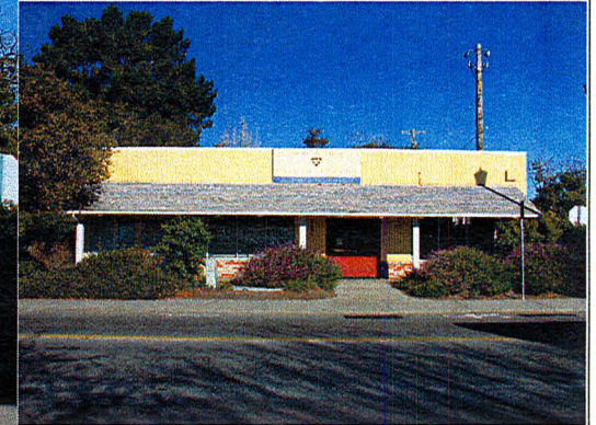
EXISTING SIGN 4'X10' WILL BE REMOVED
