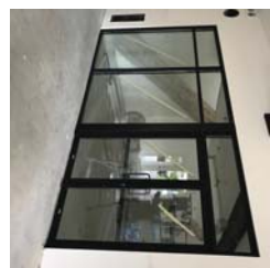
2 (N) DARK-BRONZE ANODIZED ALUMINUM STOREFRONT SYSTEM
