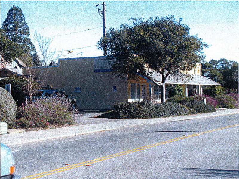
EXISTING SIGN 4'X10' ON OPPOSITE WALL WILL BE REMOVED
