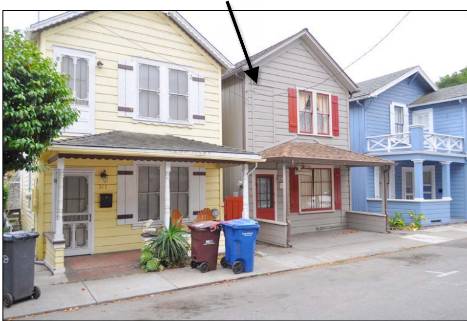
Figure 2. Current image of the Vernacular-style boarding houses on Cherry Avenue. The central building is the subject property. Note the upper-floor entry doors on the left side of the buildings, with the opening on the subject property enclosed with wood siding (arrow).
