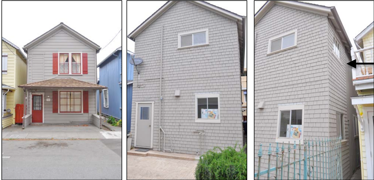
Figures 3 - 5. Left image shows the front (north) elevation, as viewed from the street. Center image shows the rear elevation, with circa-1930s rear addition clad in shingles. Right image details the rear and left side elevations, showing the border between the original wall and rear addition with an arrow.
