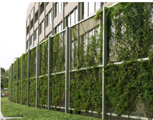
Example of espalier with vertical landscaping providing screening of blank wall area.
