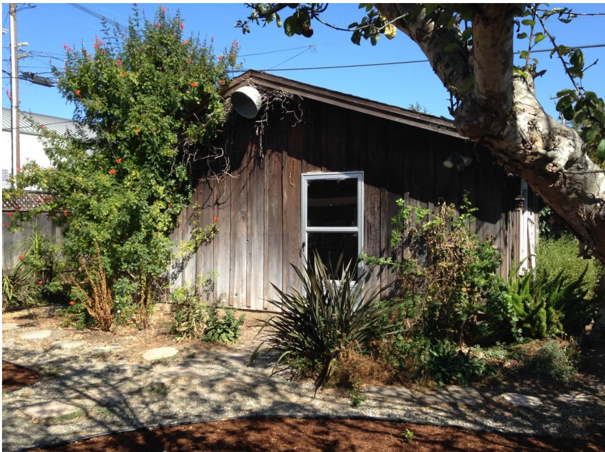
Rear view of existing garage at 416 Monterey
