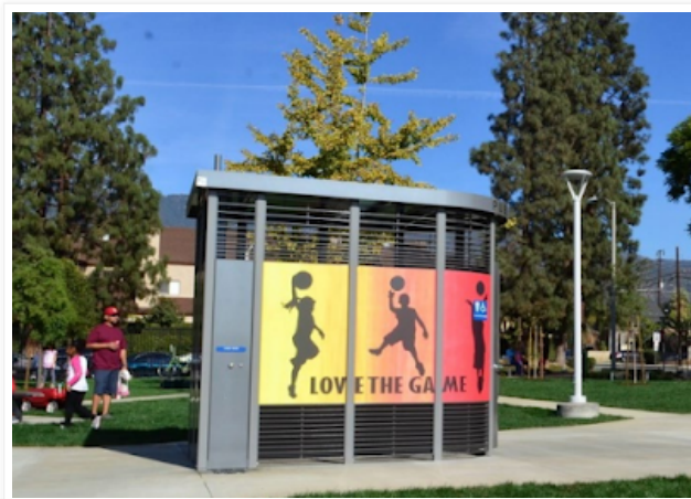
Example of toilet that will go in Library Park.
