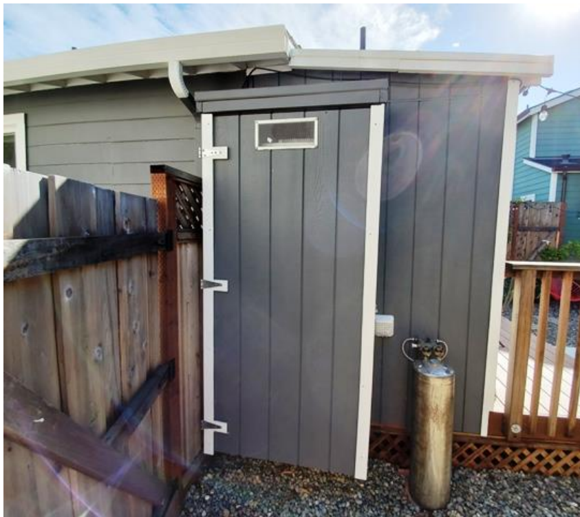
Utility Addition to Southwest Corner of House. Viewed facing east. May 2020. (Photo by Matthew Orbach, City of Capitola)
