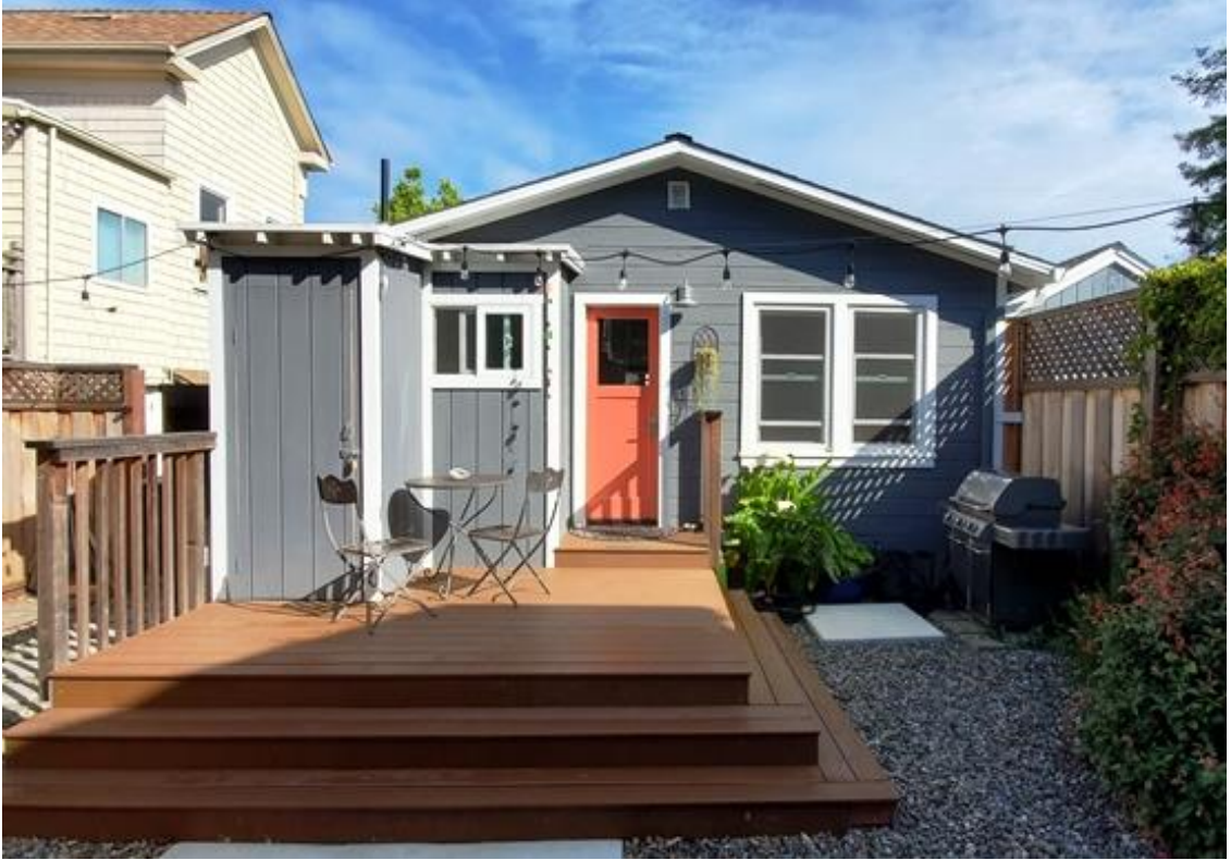
Rear Elevation. Viewed facing north. Indicates utility addition and altered paired window unit. May 2020. (Photo by Matthew Orbach, City of Capitola)
