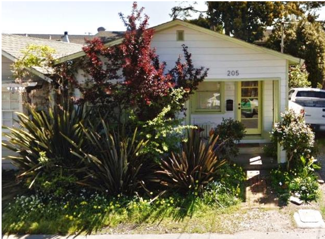
Front Façade prior to renovations. Viewed facing south. Documenting original house details. (Photo taken from Google Streetview, Accessed May 2020)
