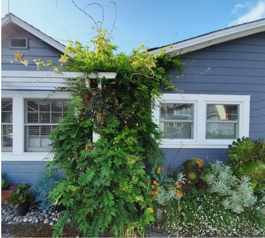
Detail of Front of House. Viewed facing south. Showing proximity to neighboring cottage. May 2020. (Photo by Matthew Orbach, City of Capitola)
