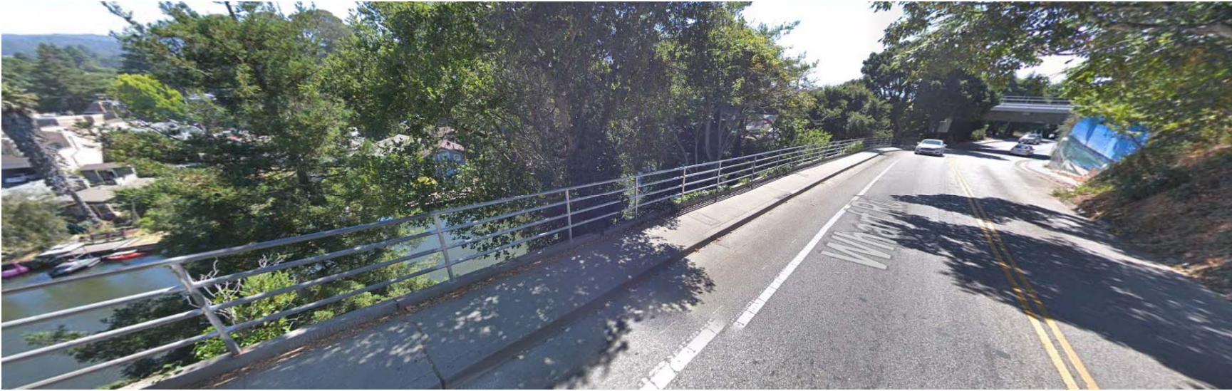
1 Capitola Road Railing
