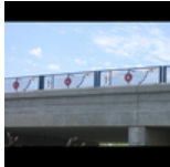
Trinity Parkway Bridge, detail
