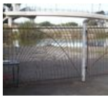
Aquatic Park Fence and Gates mild steel 6" x 90" x 6" $10000.00
