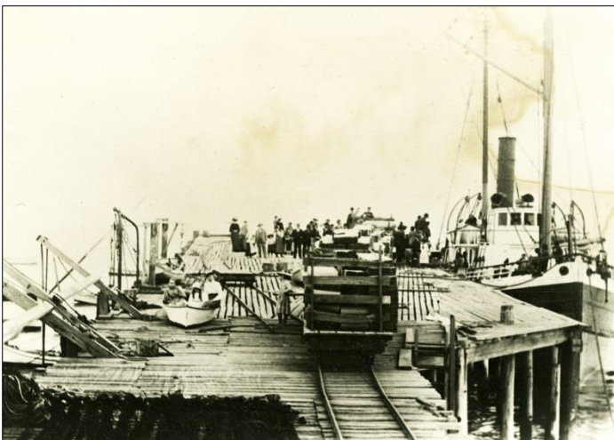
An early image of Soquel Landing shows a ship loading lumber. From Soquel, freight was transported along Wharf Road, reaching the end of the wharf on the rail car seen here. Note the fishing boat davits to the left & the people sitting in the row boat hamming it up for the camera.
