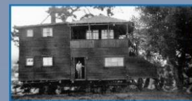
Brad Macdonald is along for the ride. He is standing in the doorway as the house is rolled into place.
