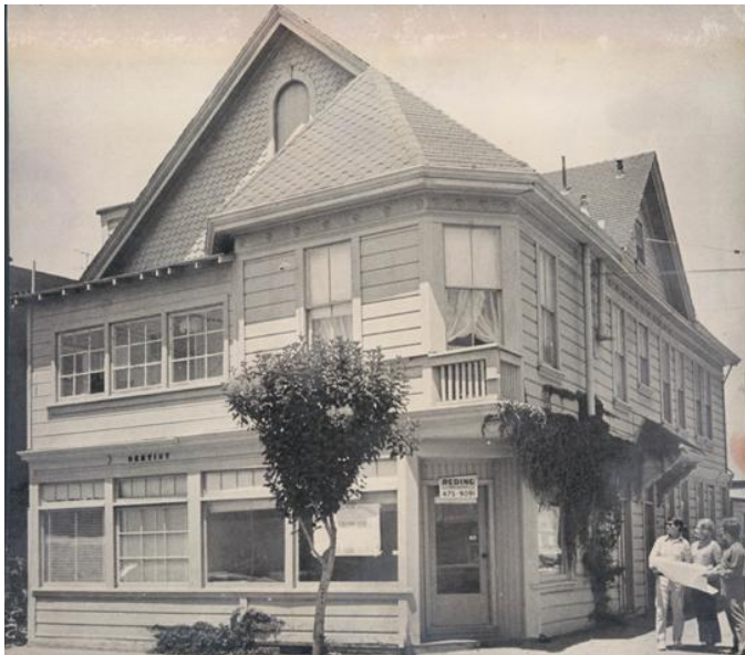
Jim and Barbara Reding look over plans for the Hihn Superintendent's Office as the 1972 renovation gets underway
