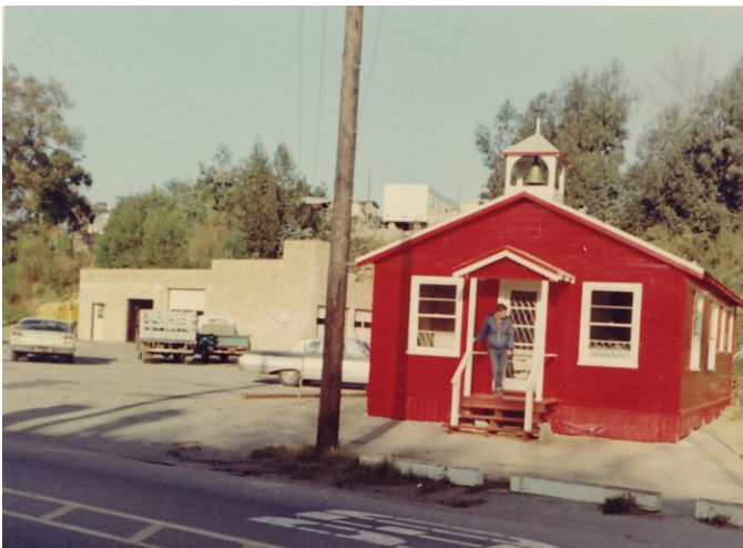
Phil Walker outside the Capitola Museum just after completion in 1967. Note the old city corporation yard to the left, where City Hall is today.
