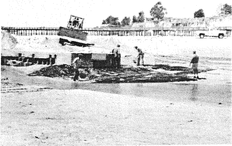
Plastic Sheeting, Flume Entrance
