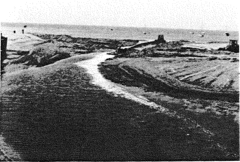
Sandbar Construction 16May91
