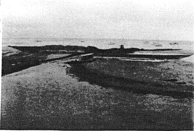
Sandbar Construction 15May91
