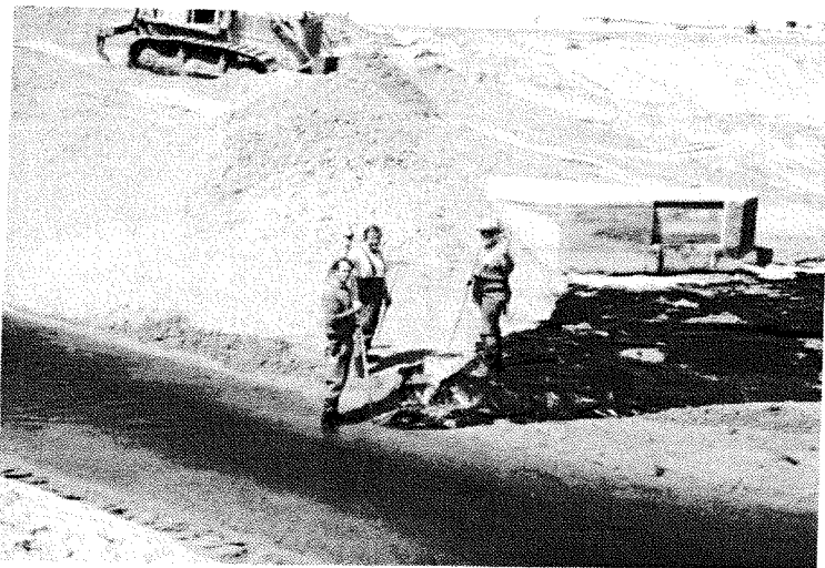
Covering the Flume 20May92
