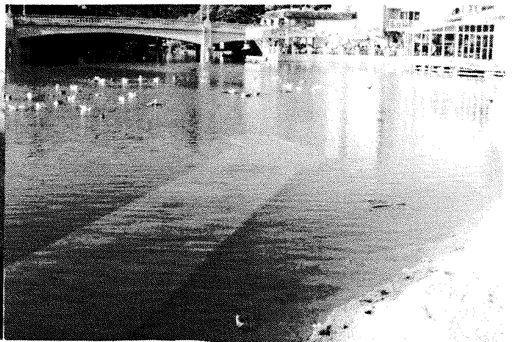
Submerged Flume @ High Tide 13Nov92
