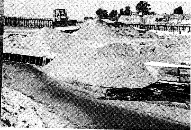
Covering the Flume 20May92
