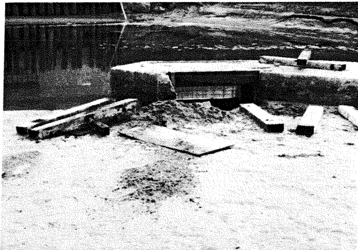
Preparing Flume Entrance 18May
