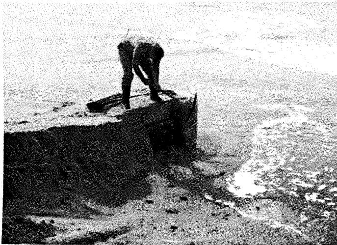
Opening the Flume Exit 18May93
