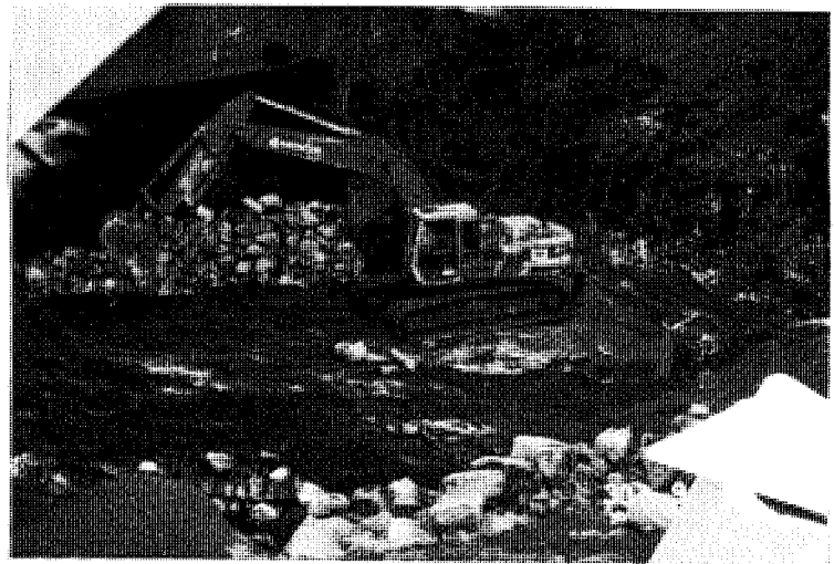
Rip-rap Placement Under Porter St. Bridge, 30Sep94
