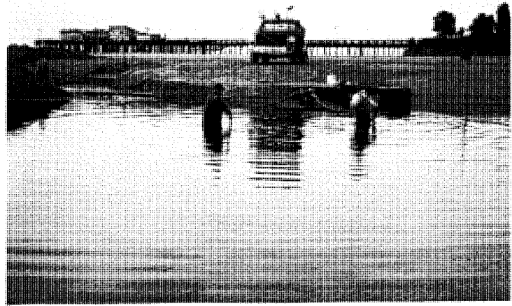
Raking and Flushing of the Flume 17May94
