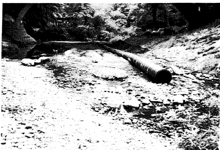
Culvert Impassable @ Hwy 1, 30Jul94
