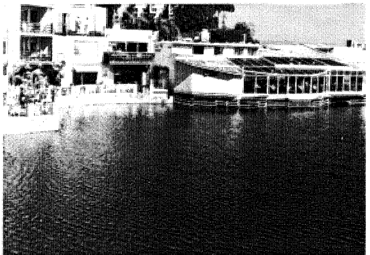
Reach 1, Restaurant Cove 12Sep95
