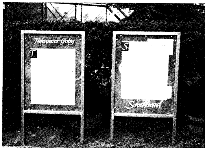
Refurbished Signs with Stainless- Steel Frames and New Lexan Covers 4Feb96
