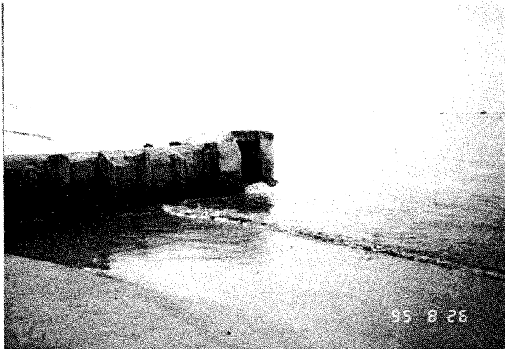
Flume Exit Passable 26Aug95
