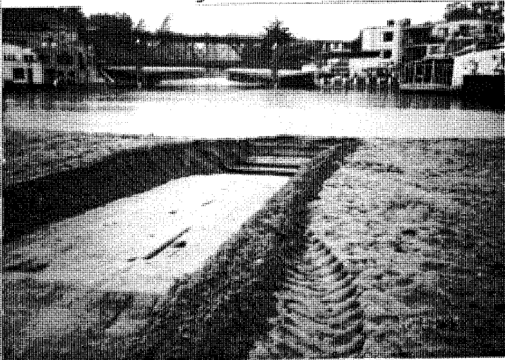
Notch Ready for Potential Sandbar Breach 11Dec95
