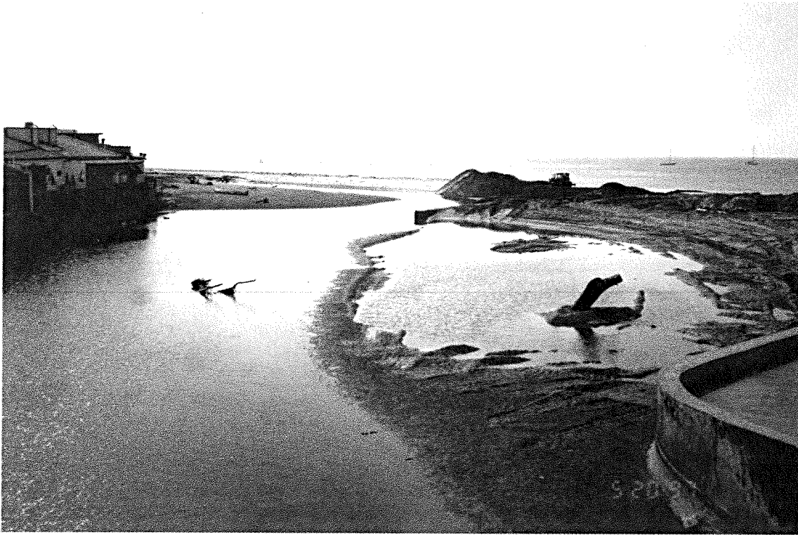
Estuary Showing Excavated Area on Right, Lateral Channel Across Beach and Stock-piling of Sand for Blockage, 20May97
