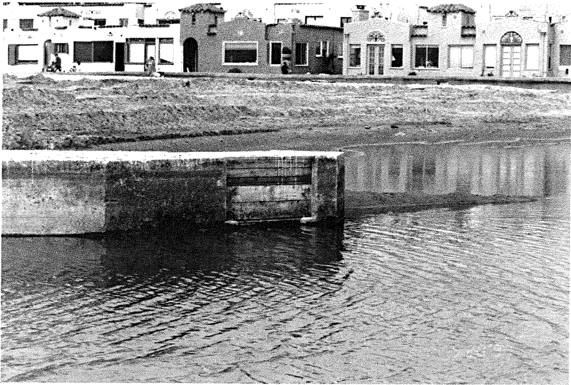
Flume Inlet Before Sandbar Construction Began, 20May97
