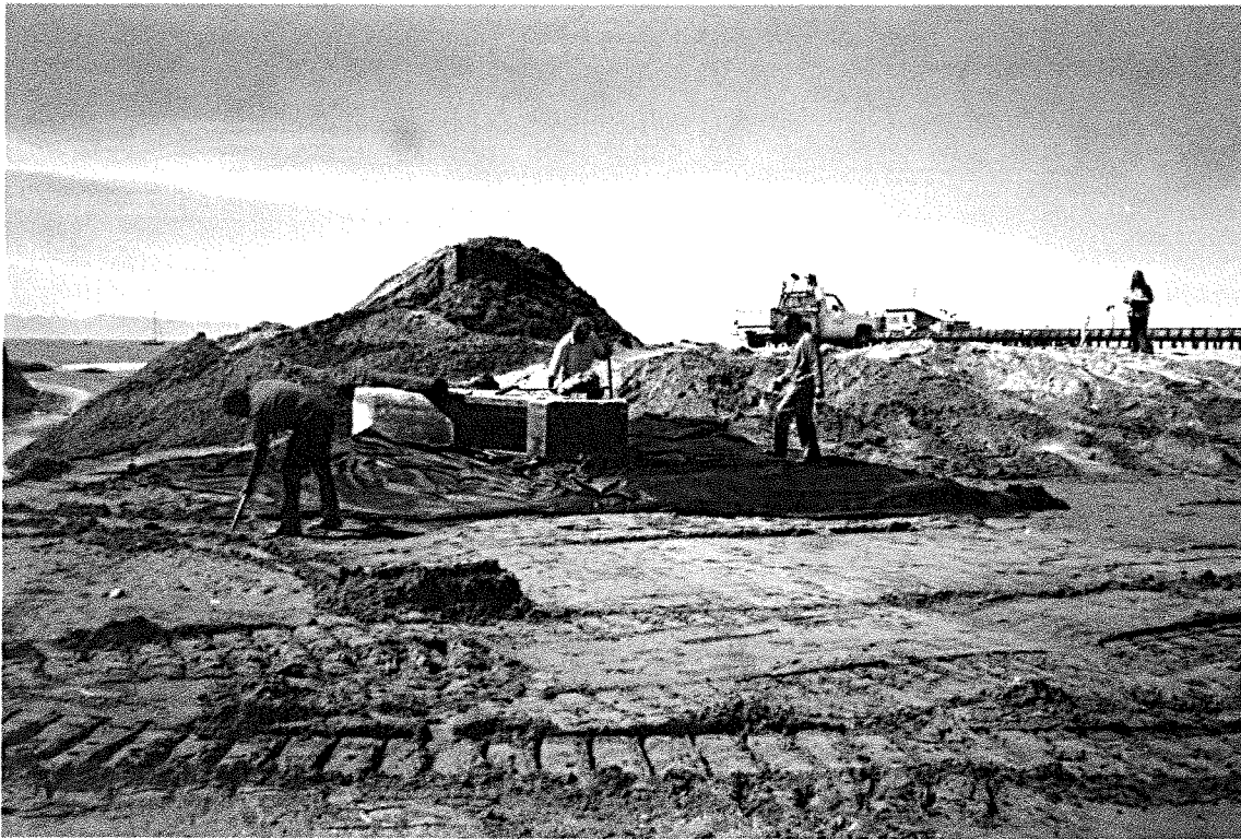
City Staff Spreading Geo-fabric Over Visquine Around Flume Entrance, 27May97
