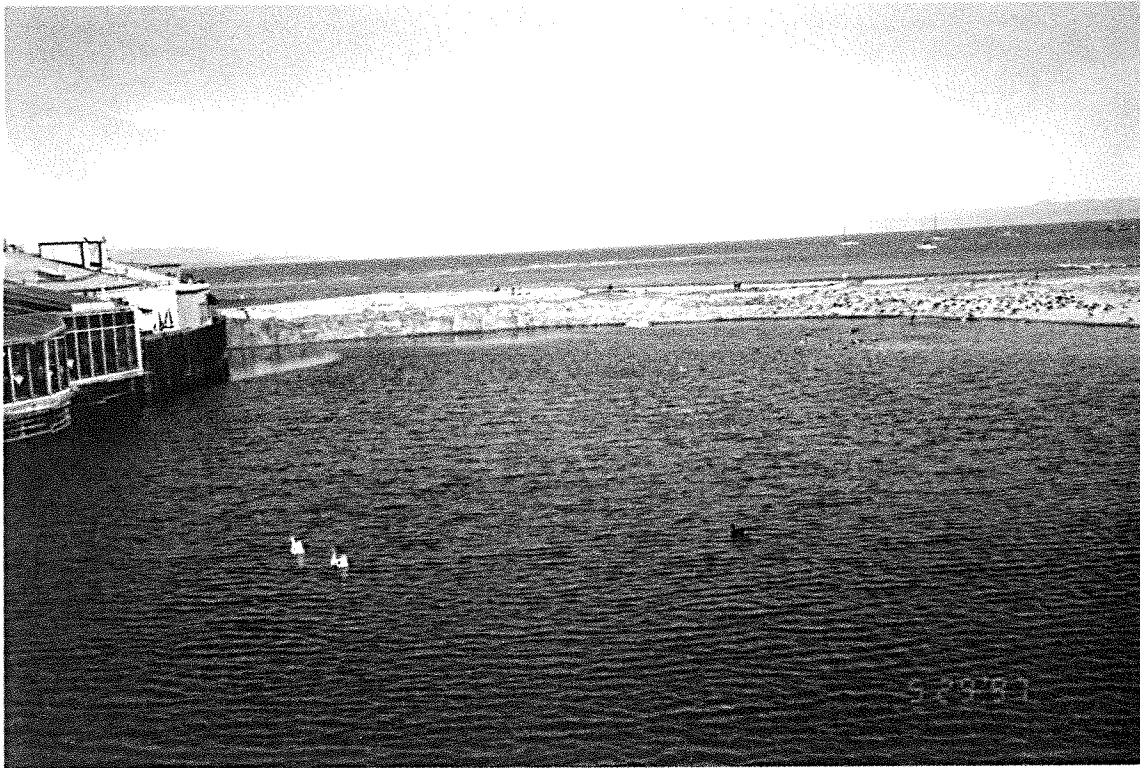
Lower Lagoon after Sandbar Construction, 29May97
