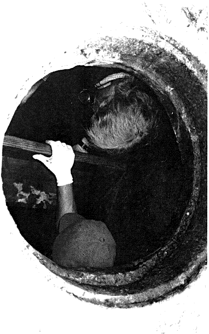
Baffle Being Installed Inside the Flume by Ed Morrison, 22May97
