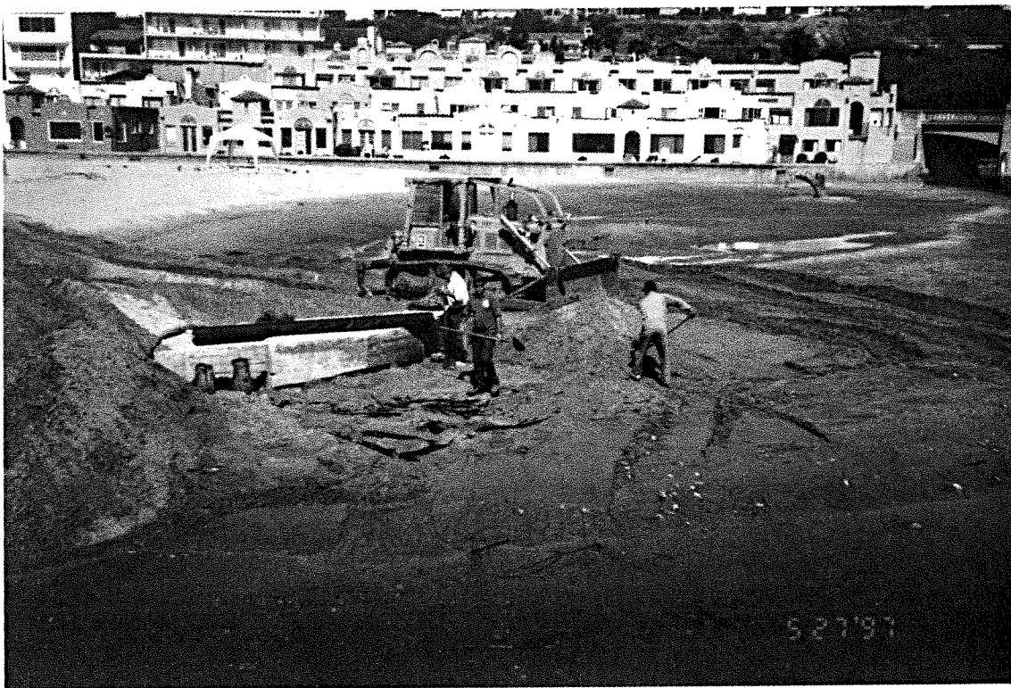
City Staff and Equipment Operator, Bill Casalegno, Covering Geo-fabric With Sand, 27May97
