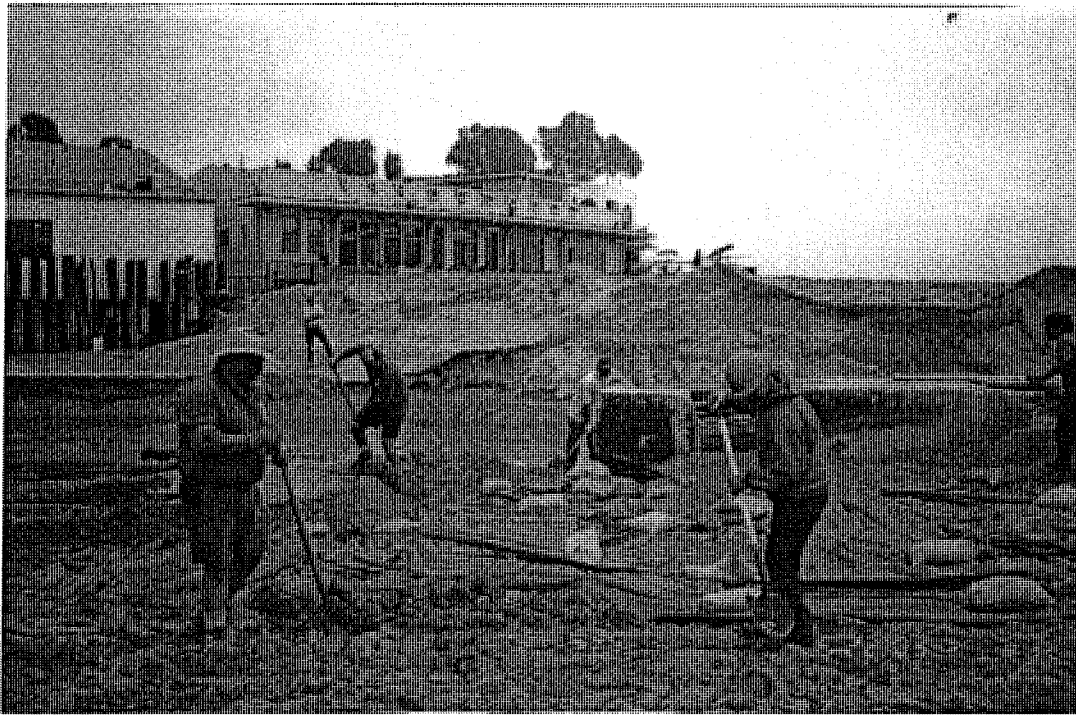
Preparation of the Flume Inlet Prior to Lagoon Closure
