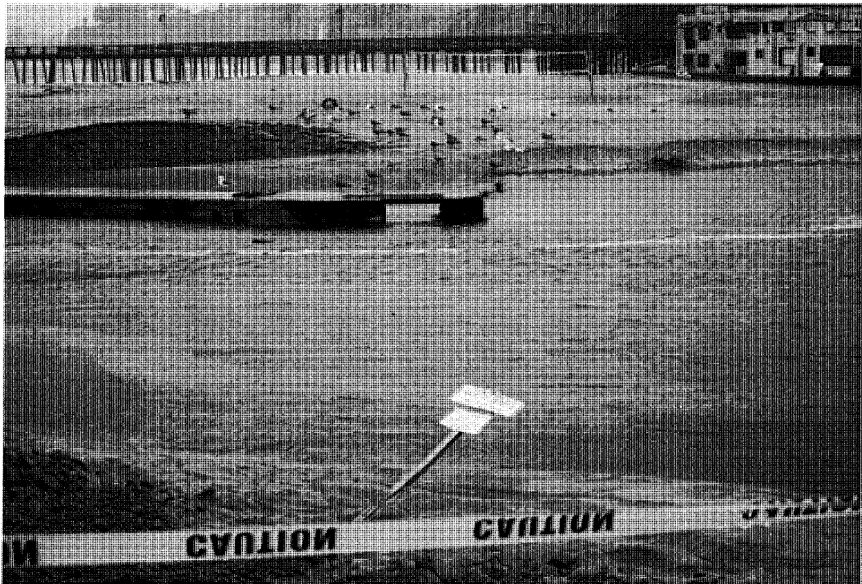
All Boards Had Been Removed from Flume Inlet to Maximize Flume Capacity Prior to Breach 19 October 2004
