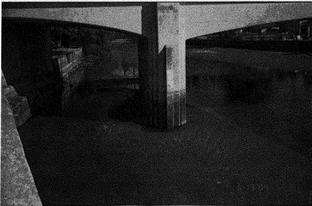
Normal Soquel Creek Estuary Under Stockton Avenue Bridge Prior to Sandbar Construction 19 May 2004
