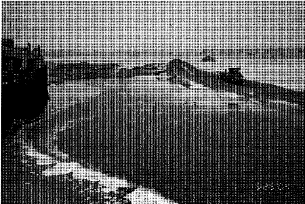
Sandbar Closed at End of Day 25 May 2004
