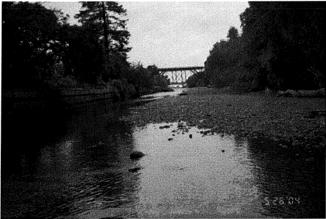
Upper Reach 3, Looking Downstream Toward Trestle at Low Tide 26 May 2004
