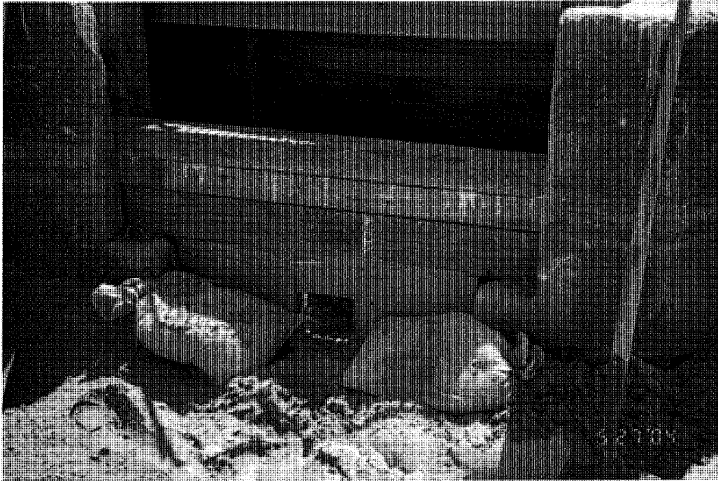
Underwater Portal for Adult Steelhead Passage Through Flume Inlet 26 May 2004 (Film Date Incorrect)
