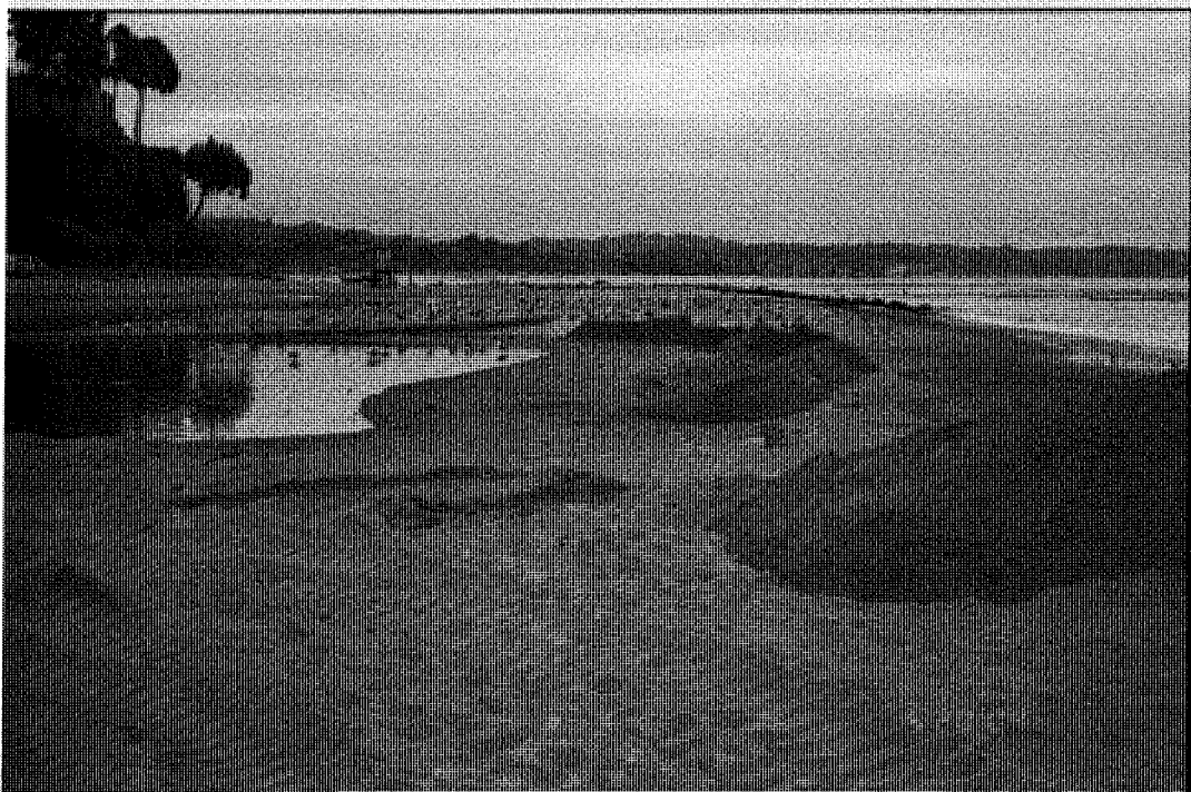
Precautionary Berm to Maintain High Water Level in Lagoon for Flushing of the Flume 20 May 2004
