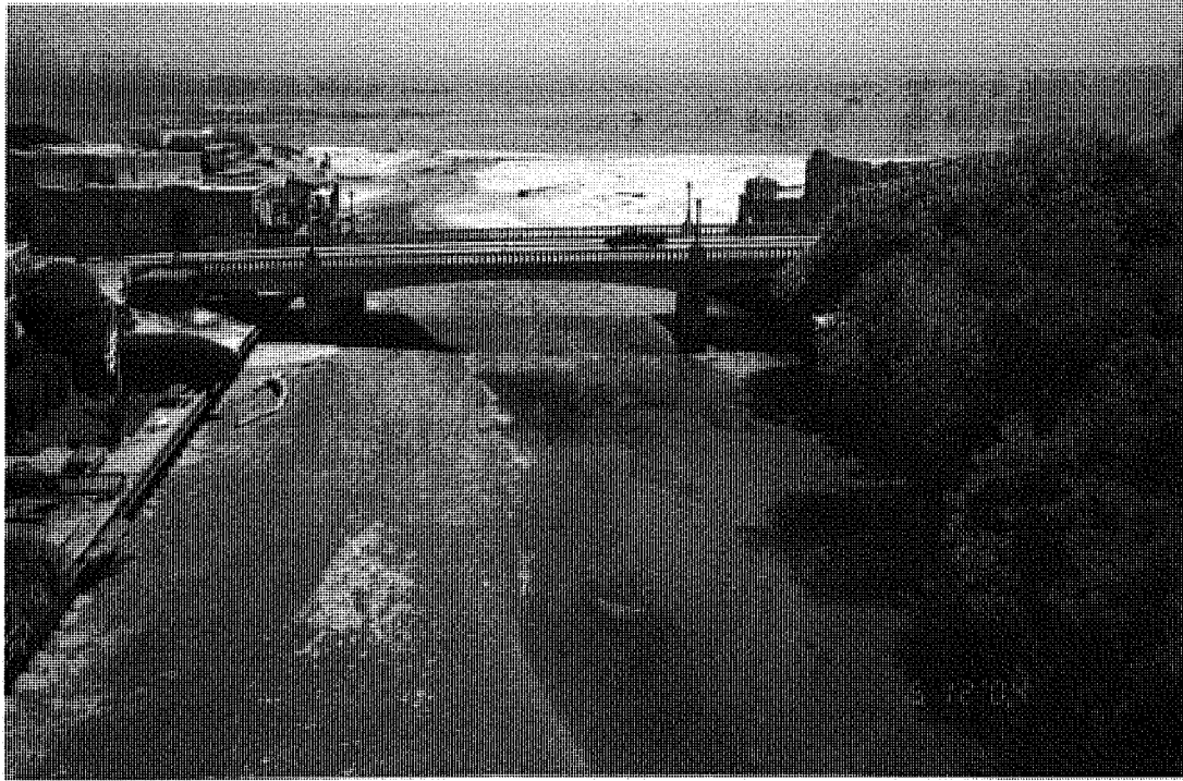
Normally Functioning Soquel Creek Estuary, Looking Downstream from Trestle 12 May 2004
