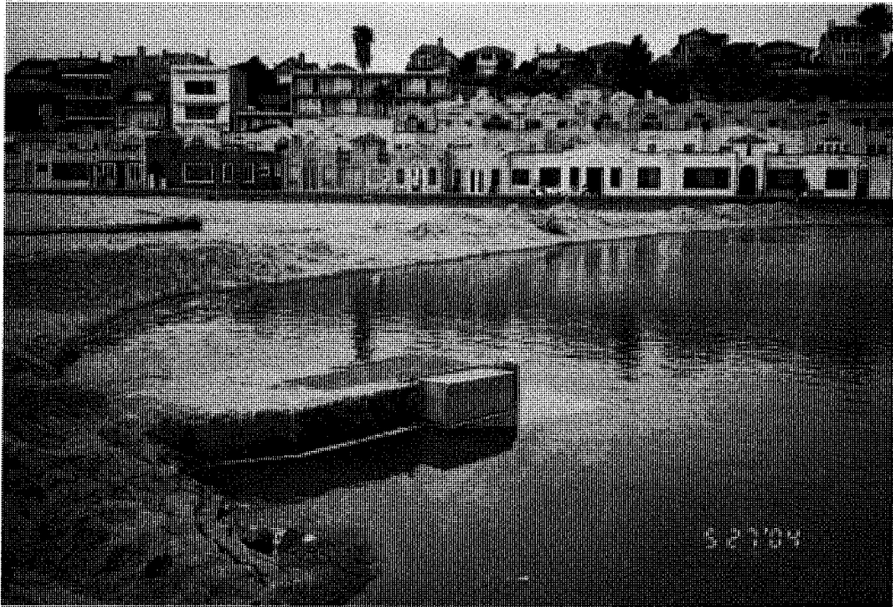
Shroud Placed on Flume Inlet after Saltwater was Detected in Lagoon 27 May 2004
