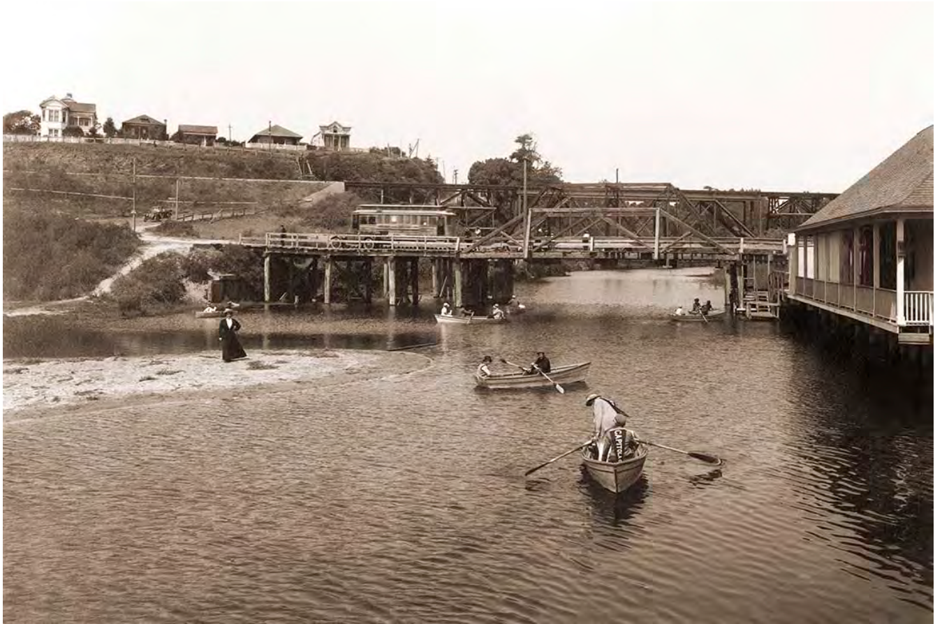
Later Wooden Stockton Avenue Bridge with adjacent Trolley car bridge and wider lagoon under western bridge portion and in later Venetian Court location (Railroad Trestle free-spanning the stream channel further upstream); circa 1910 (Courtesy of the Capitola Historical Museum)
