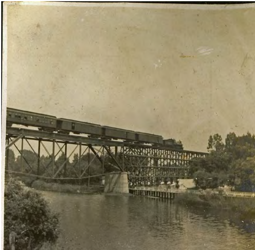
Soquel Lagoon- East margin with Boardwalk, tule marsh and later steel, free-span Railroad Trestle with concrete abutments; circa 1920 (Courtesy of the Capitola Historical Museum)
