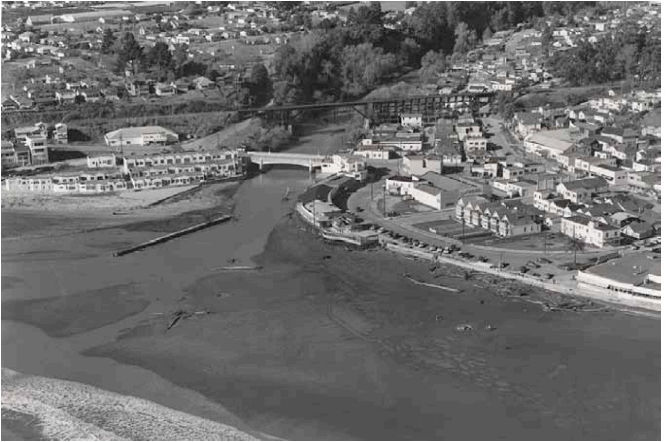
Post-World War II Soquel Creek Estuary at very low tide- present-day Stockton Bridge with flume exposed on the beach after the December 1955 flood. Riparian corridor re-established on west side above Stockton Bridge; circa 1955-56 after the flood (Courtesy of the Capitola Historical Museum)
