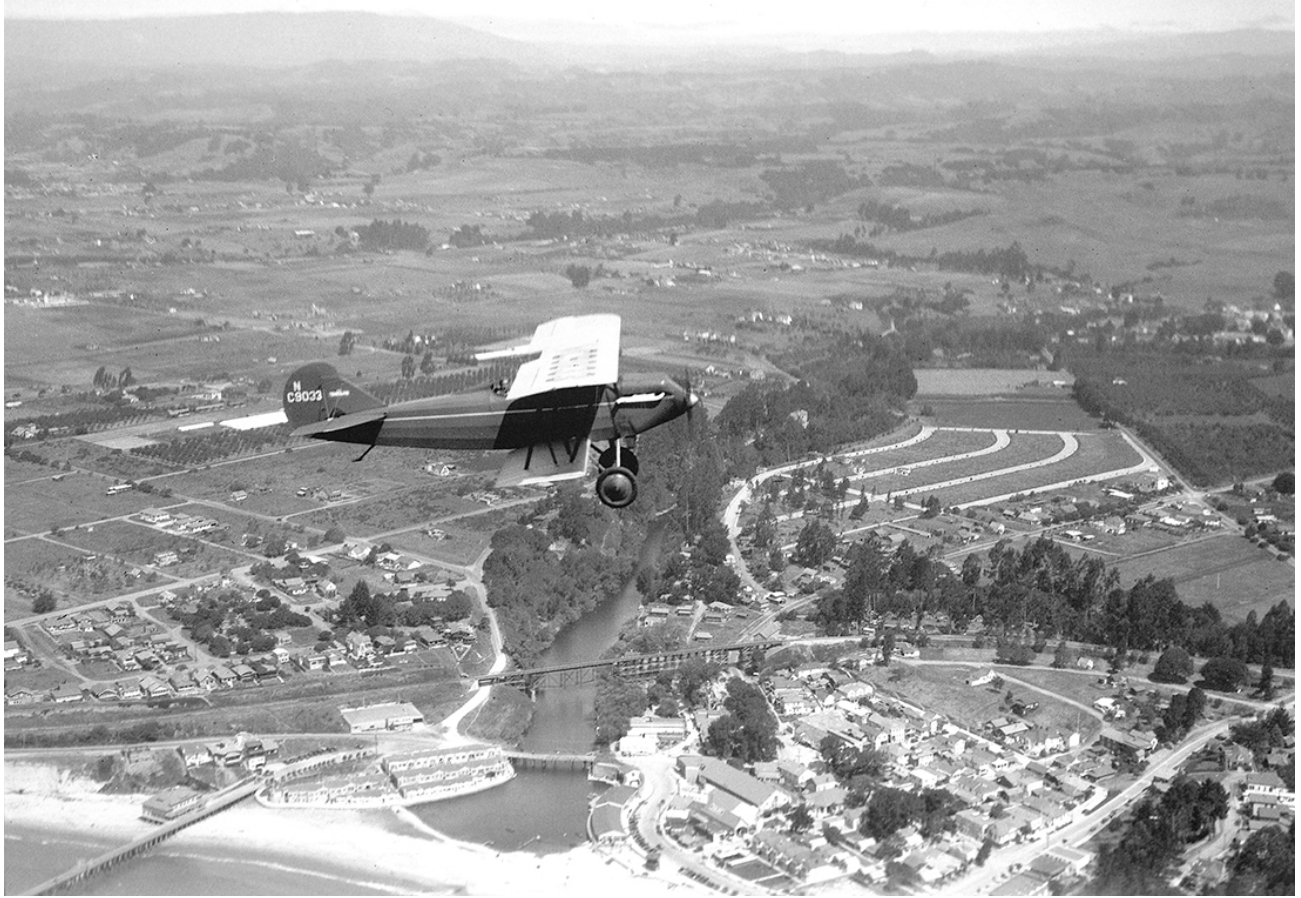
Soquel Lagoon Post-Venetian Court Construction- Older Stockton Avenue Bridge and prior to expanded development on eastern margin of the Lagoon, above and below the Railroad Trestle; circa 1931. (Courtesy of the Capitola Historical Museum)
